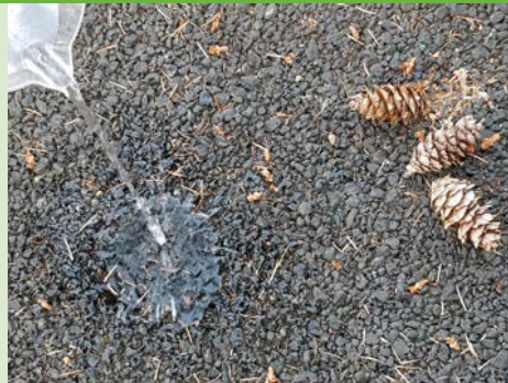
Water poured on permeable pavement quickly soaks in.
